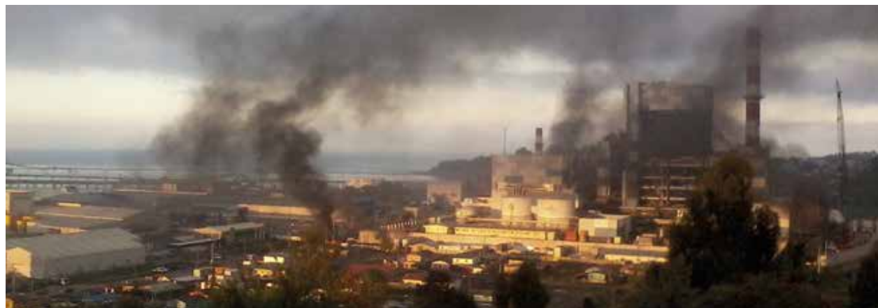
Photograph: Ventanas Power Plant, Puchuncaví / Source: Chile Sustentable.
